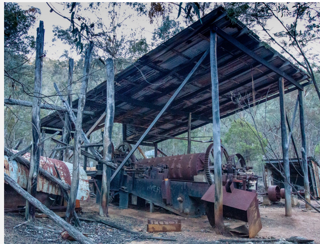
Historic Cassilis mine surface works
